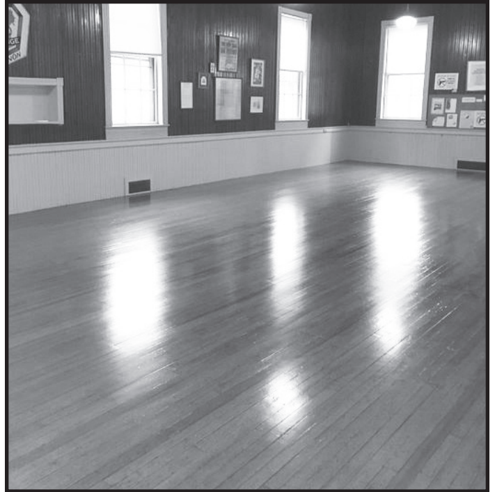
The floors at Cannon Grange No. 159 have been sanded and refinished, bringing them back to their original beauty.
